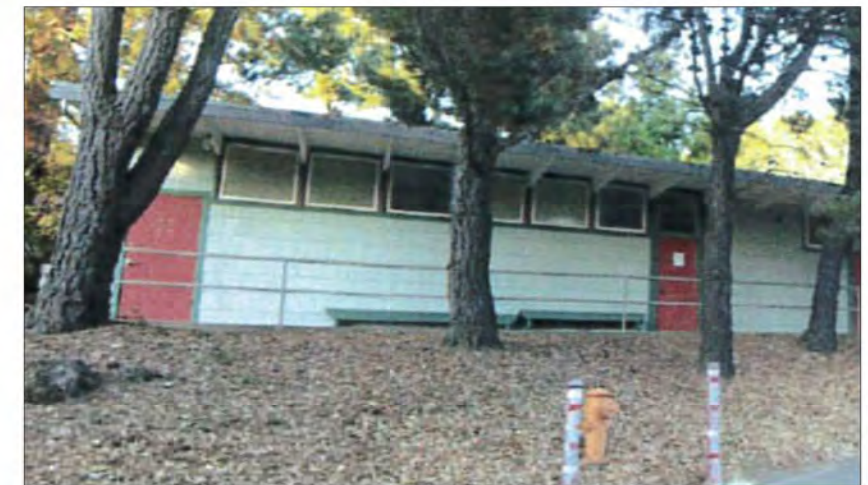
SITE 2: ANNEX BUILDING
