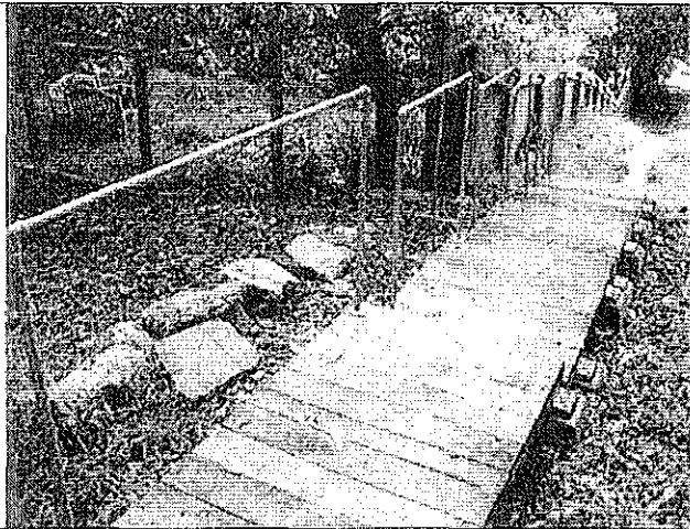
Fig. 8: One segment of the Glendale Path is constructed with planks supported by timber girders atop small concrete piers. The slope in this area is not steep enough to warrant a stairway but is sufficiently large to make standard sidewalk-style paving impractical.
