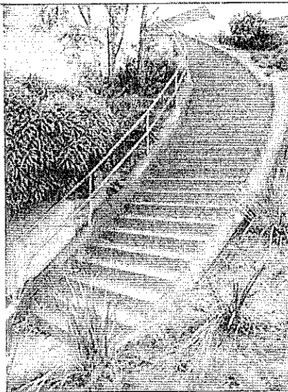
Fig. 2: San Francisco's 12 th Avenue steps are curved to connect a Y-intersection.
