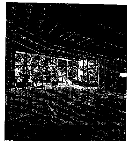
Esalen Lodge Renovation Under Construction
