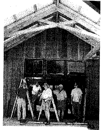
Arastradero under construction, Palo Alto, CA
