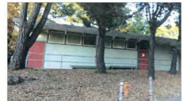
SITE 2: ANNEX BUILDING
