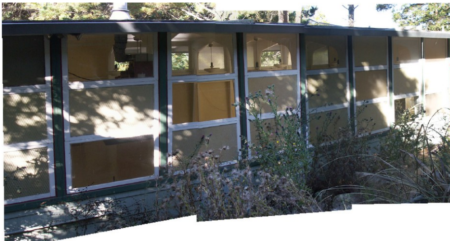
Below: View from the back yard, showing variety of types of glazing.
