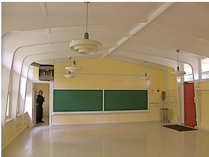
Annex interior, with painted wood arches. Large windows face east; high windows face the covered walkway.
