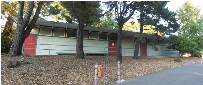
Front of Annex with covered porch, as seen from parking lot.
