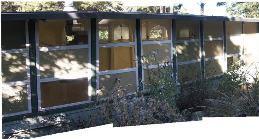
Below: View from the back yard, showing variety of types of glazing.
