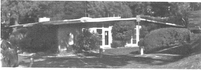
Above: Community Center exterior.
